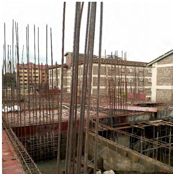
Form work complete.
