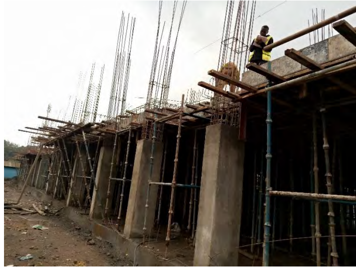
-Form work already complete.
