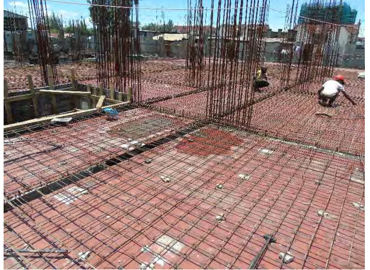
-Colum work on basement done.
