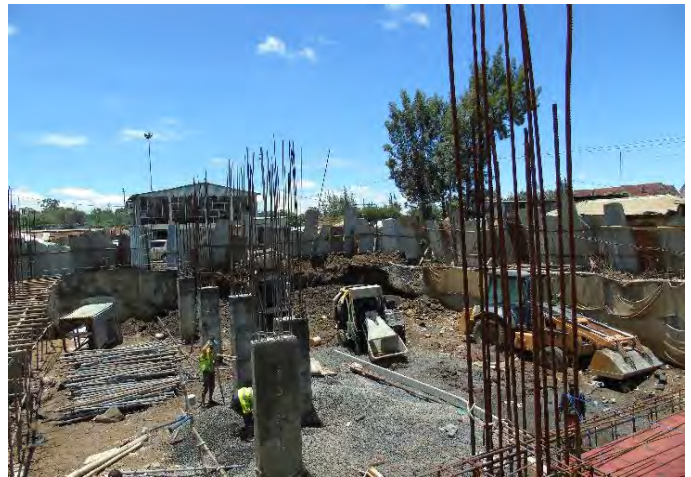
-Column casting work underway.
