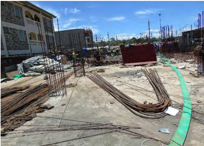
-Ground floor slab casting underway.
