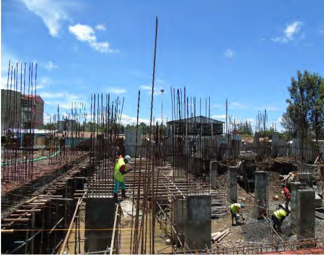
-Steel fixing on ground floor underway.
