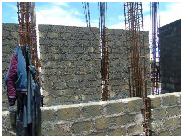
Blockwork in sections of ground floor underway
