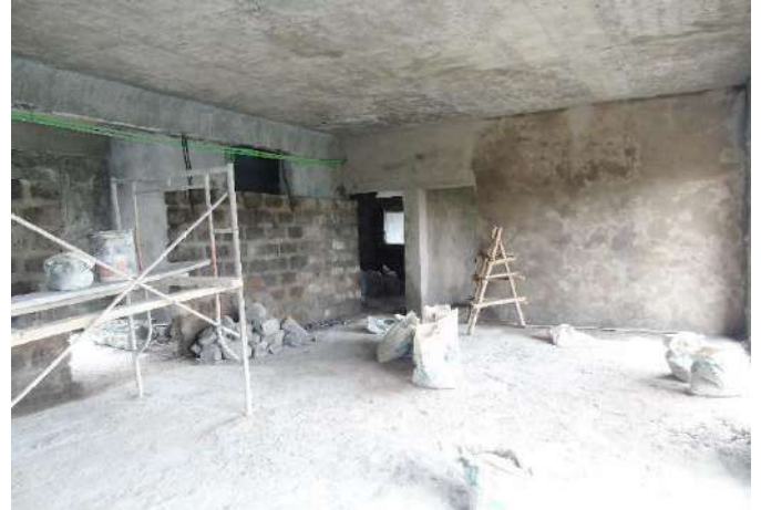
-Electrical piping & plumbing work underway.
