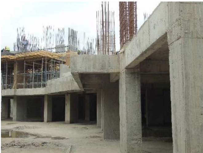
-Plastering on columns underway.
