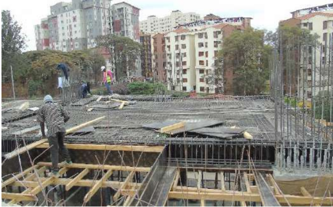
-Formwork for slab casting on 1st floor underway.
