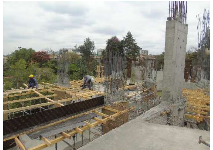
-Reinforced column concrete work underway.
