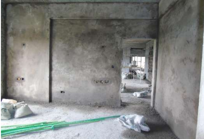
-Interior wall plastering in show house unit underway.
