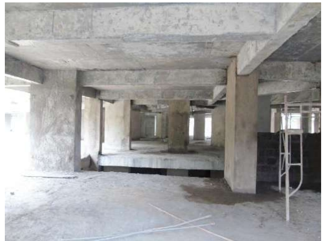
-Plastering on columns underway.
