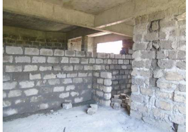
1st-Blockwork for room partitioning underway.
