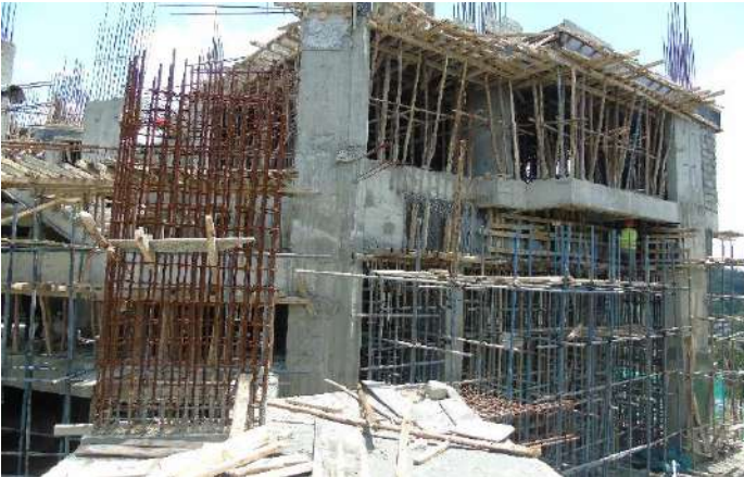
-Column casting in parts of first amenities floor done.
