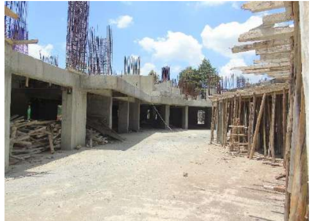
-Slab compaction in second amenities floor done.
