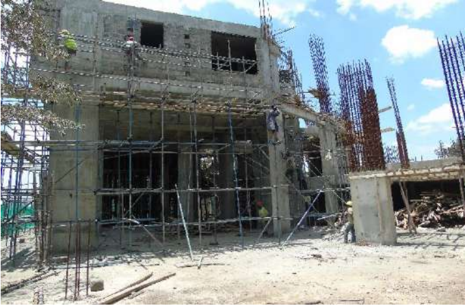
1st-Blockwork in parts of first floor underway.
