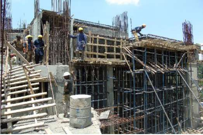
-Formwork on parts of 3 rd floor underway.
