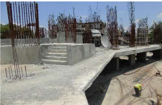
-Placement of slab reinforcement steel in parts of 2 nd floor done.
