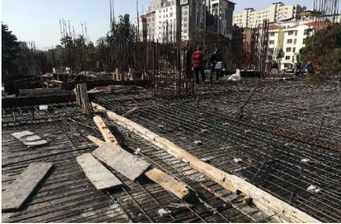
-Formwork on parts of amenities floor underway.
