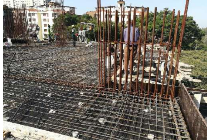
-Column & beam steel work underway.
