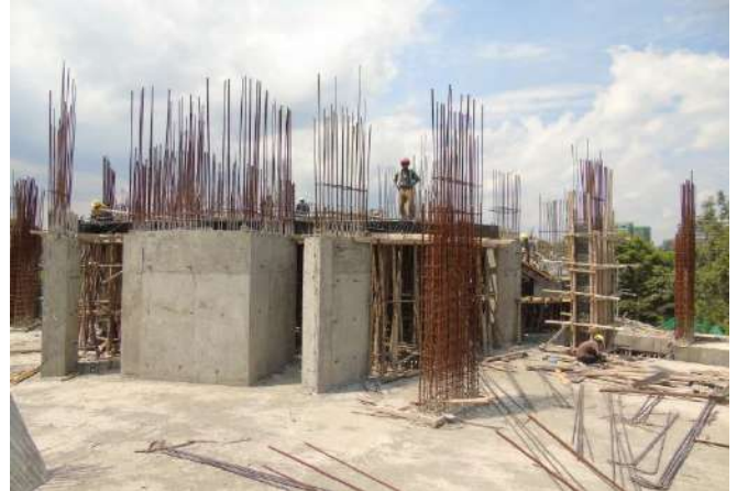
-Colum rebar work underway.
