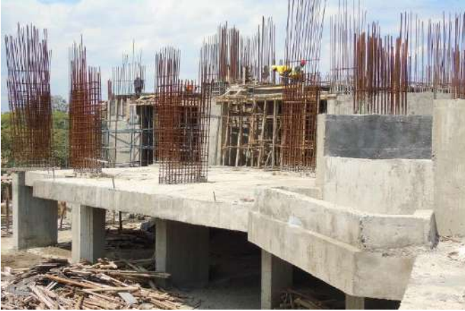
-Formwork on parts of amenities floor underway.
