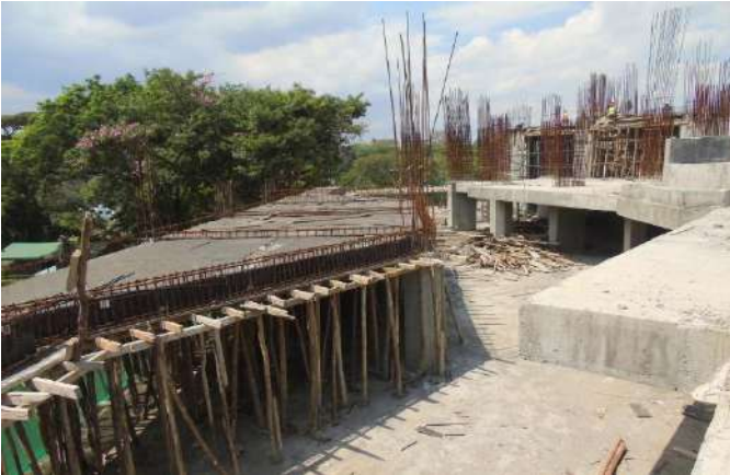
-Placement of slab reinforcement steel underway.
