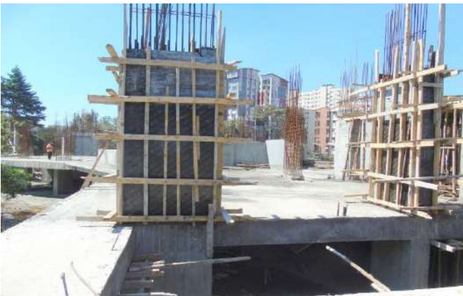
-Column casting for elevation of amenities floor done.
