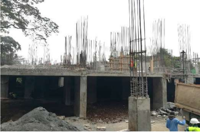
-Column rebar work for elevation of 2 nd podium floor underway.
