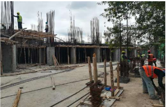
-Beam rebar work for elevation of 2 nd podium floor underway.
