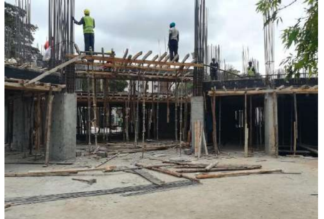
-Formwork for slab casting on parts of 2 nd podium floor underway.
