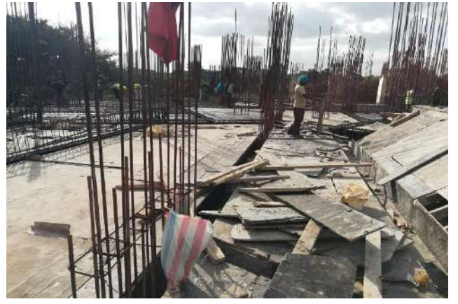
-Column & beam rebar work underway.
