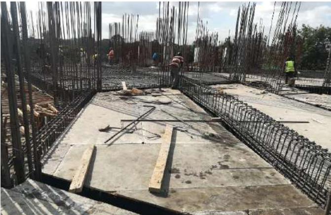
-Beam rebar work for elevation of 2 nd podium floor underway.
