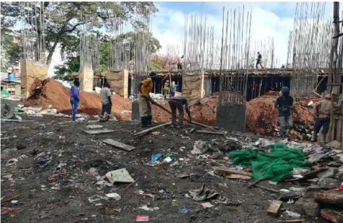
-Structural elevation work on parts of ground floor underway.
