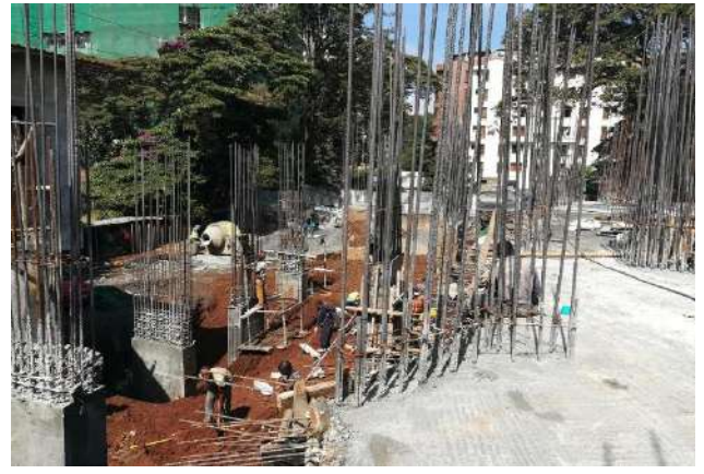
-Slab concreting on parts of ground floor underway. (basement shutter)
