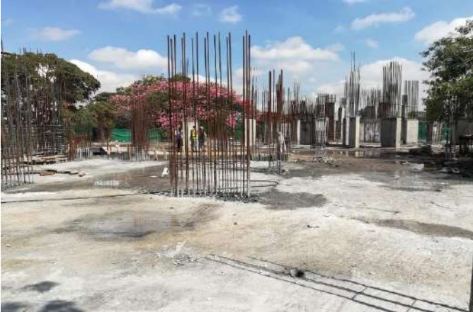
-Column rebar work on parts of 1 st floor underway.
