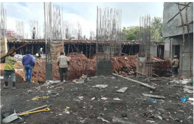
-Concreting work on stem wall done.
