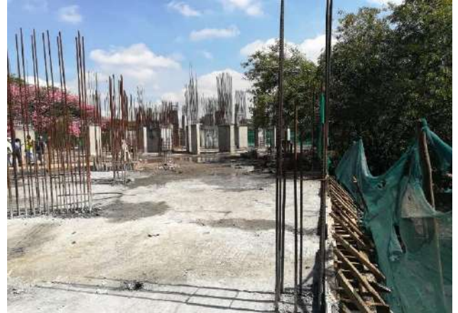
-Structural elevation work on parts of 1 st floor underway.
