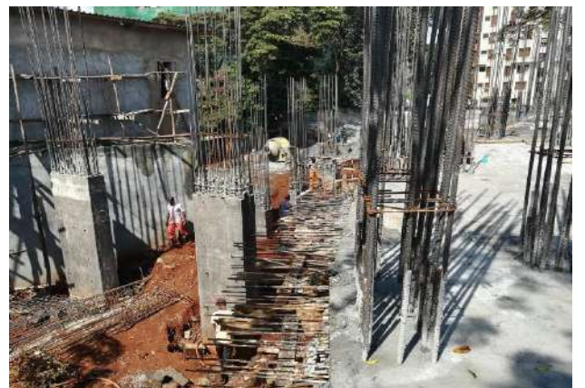
-Ground floor, Beam and column rebar concreting work underway.
