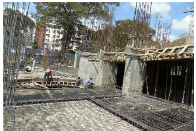
-Ground floor- Formwork, beam and column rebar work underway.
