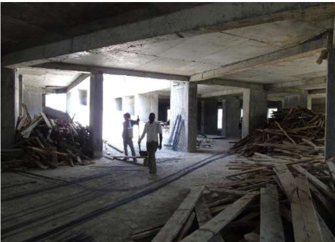
-Structural elevation work on parts of basement floor underway.
