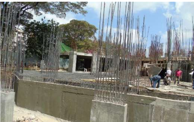
-Concreting work on stem wall underway.
