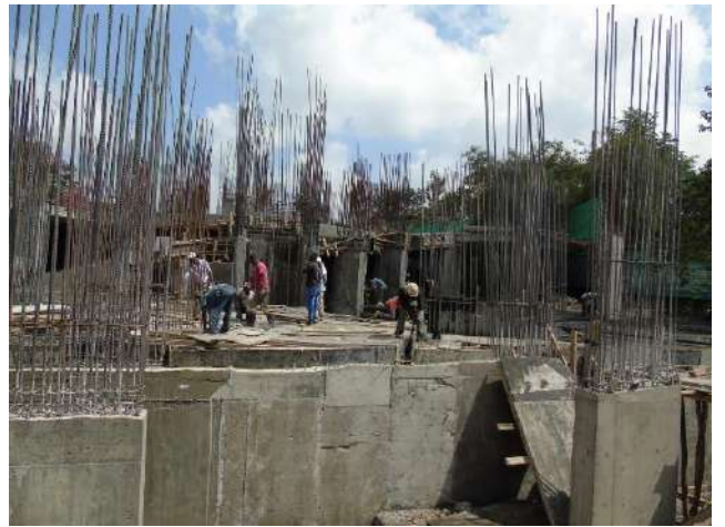
-Shuttering work on parts of basement underway.
