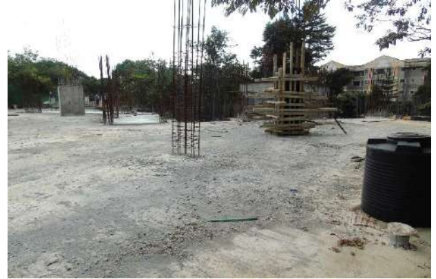
-Structural elevation work on parts of 1 st floor underway.
