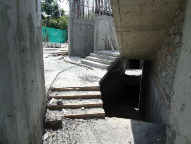
-View of basement.& ground floor.
