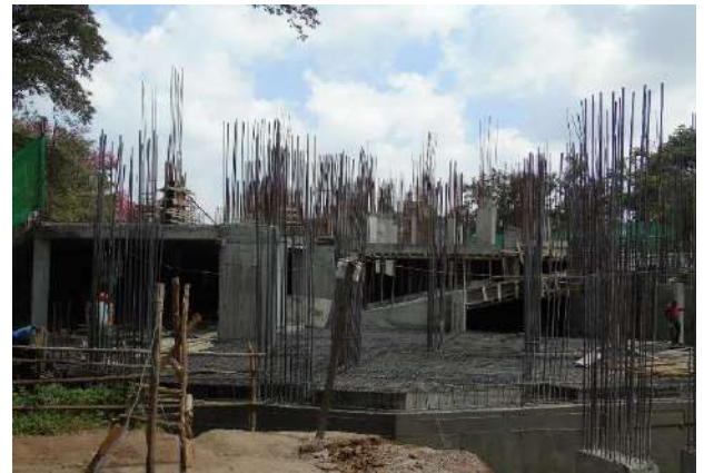
-Formwork for slab concreting on ground floor underway.(basement shutter)
