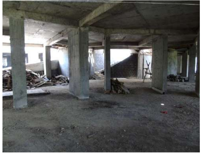
-View of basement work status.
