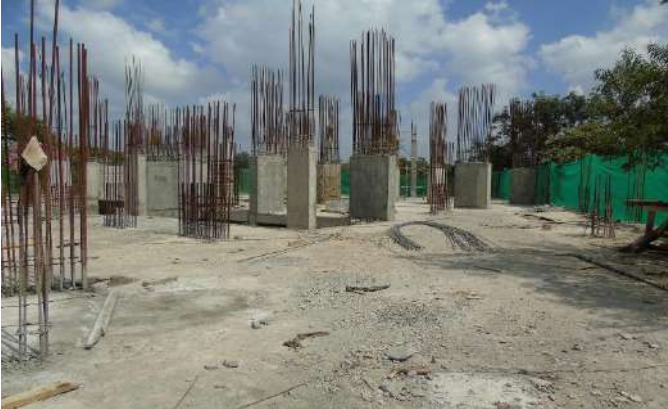
-Column rebar work on parts of 1 st floor underway.
