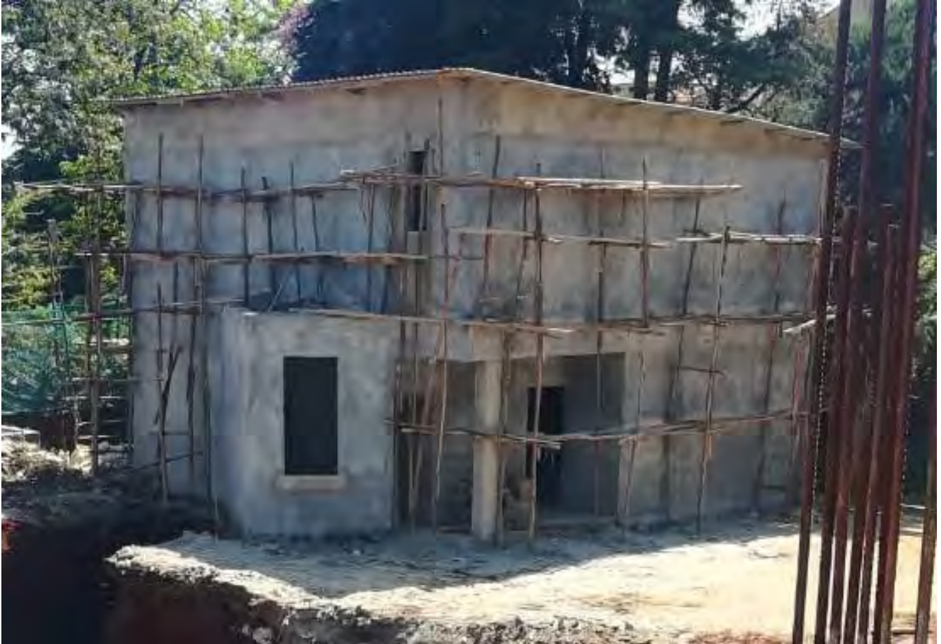
Roofing work on sample house done.
