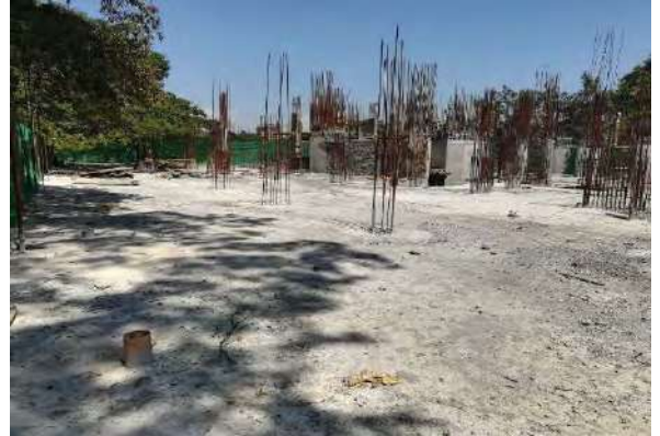
-Slab casting on ground floor done.
