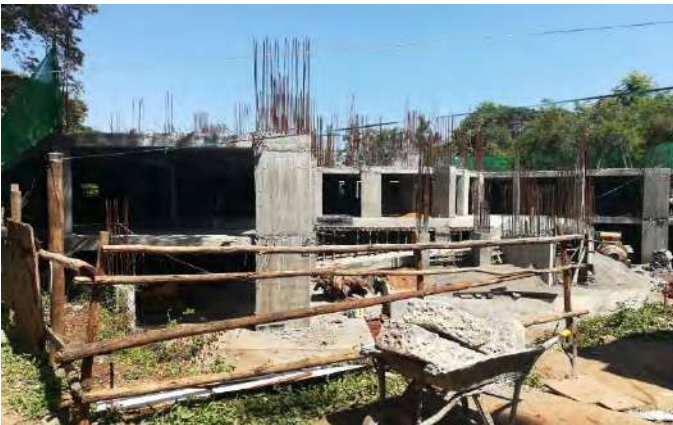
-Column rebar work on ground floor underway.
