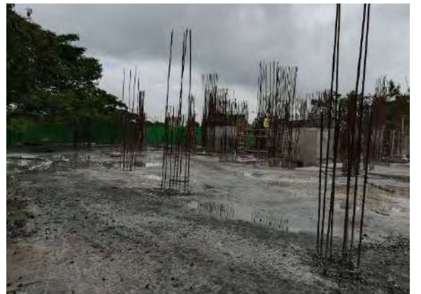
-Structural elevation work underway.
