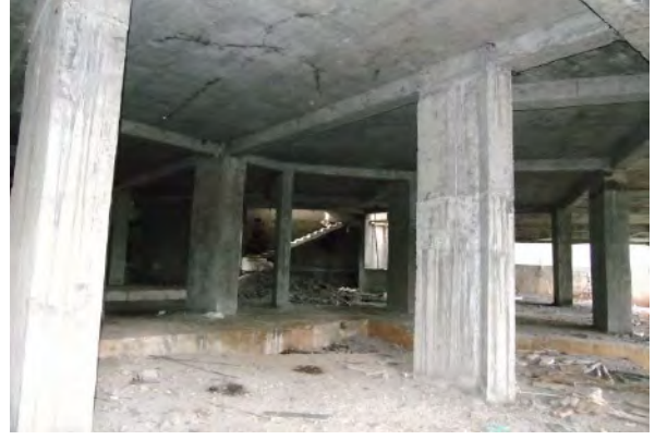
View of basement.
