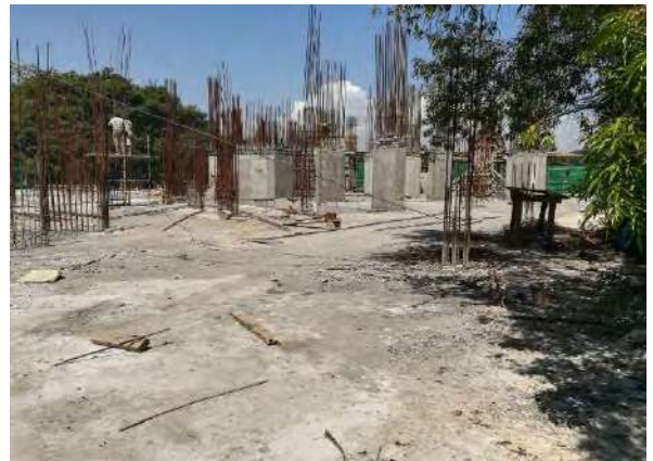
-Beam rebar work on ground floor underway.
