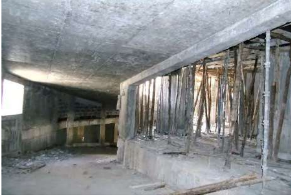
View of basement.
