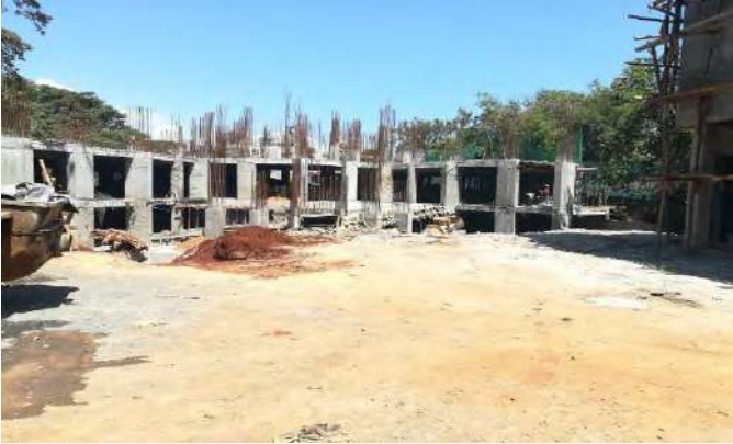
-Structural elevation work on ground floor underway.
