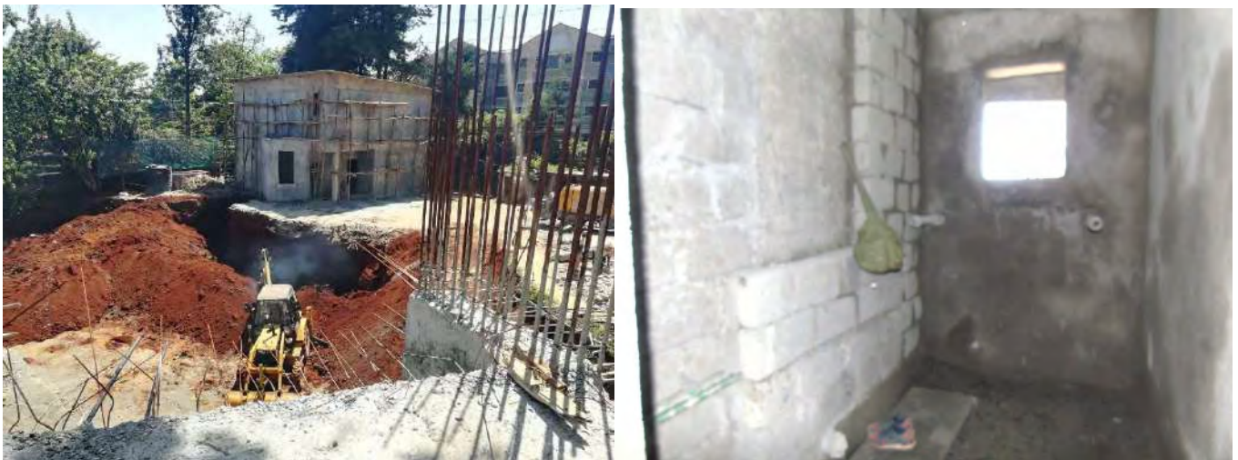
view of show house structure.
