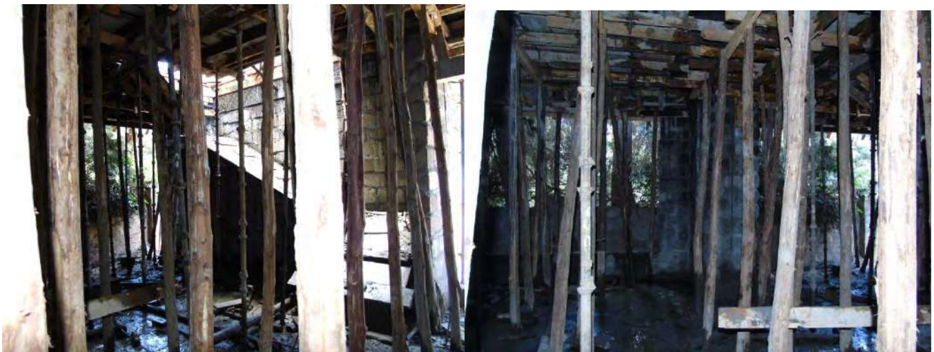
Interior view of show house structure.
