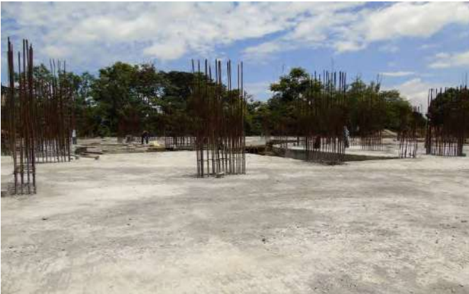
-Column rebar work on ground floor underway.
