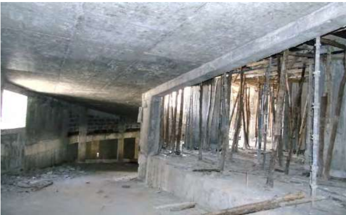
-Interior view of ground floor.
