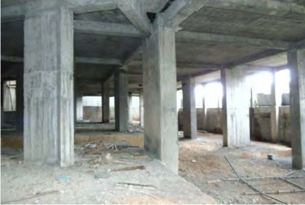
View of basement.
