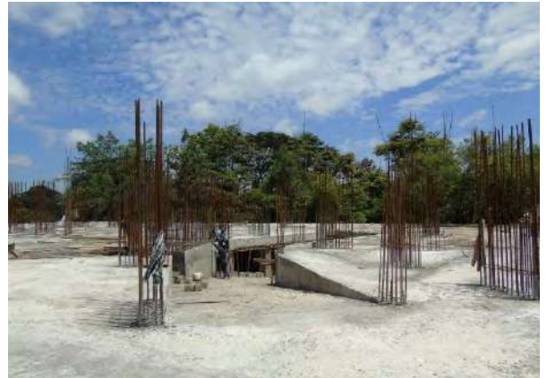
-Beam rebar work on ground floor underway.
