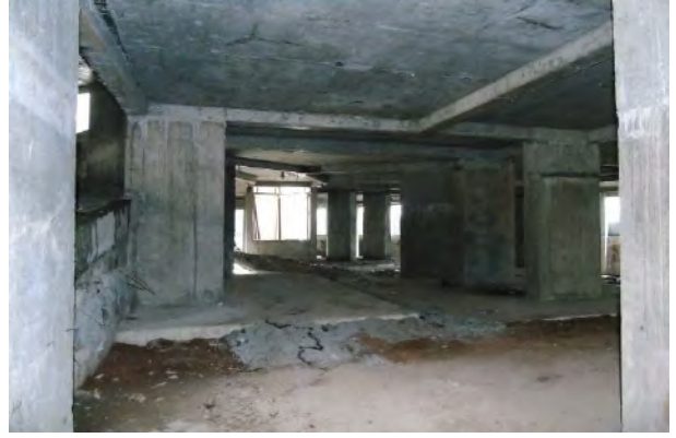
View of basement.
