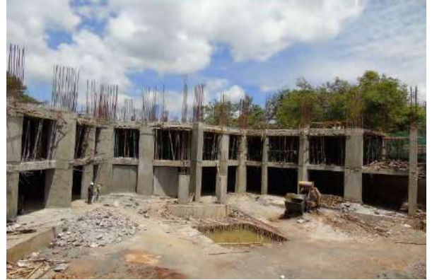
-Slab casting on ground floor done.
