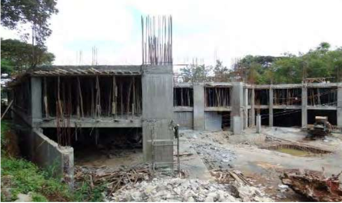
-Structural elevation work on ground floor underway.
