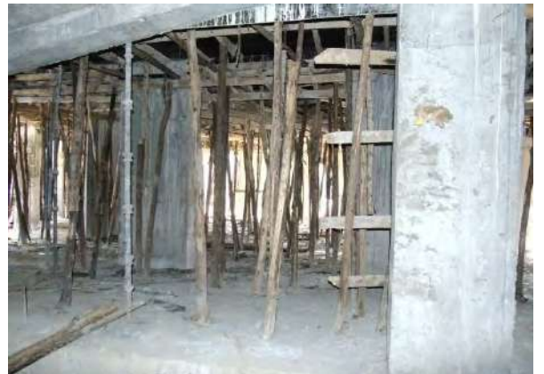
-Formwork holding on ground floor.
