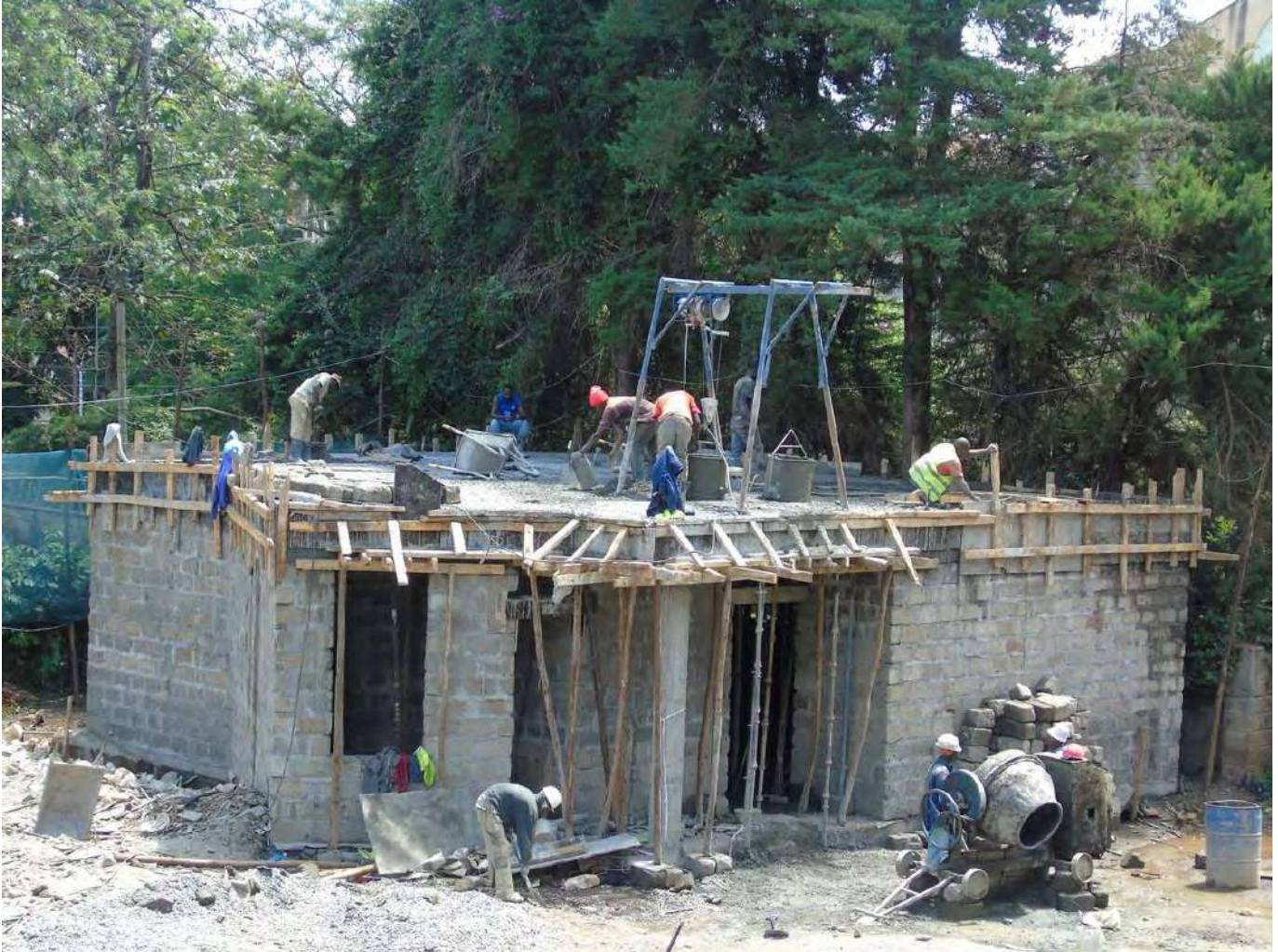
Slab Shuttering work underway.
