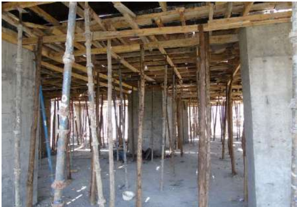
Formwork for slab shuttering on parts of ground floor underway.
