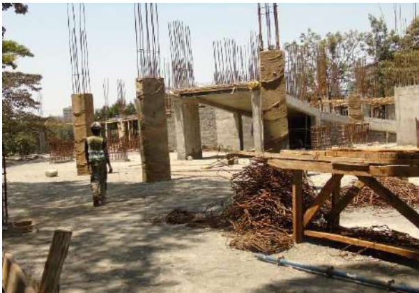
Beam reinforcement work on parts of ground floor underway.
