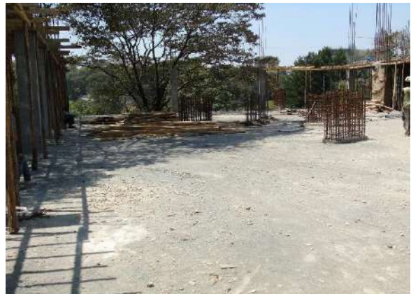
Column rebar work on ground floor underway.
