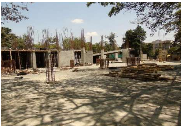
Formwork on sections of ground floor underway.
