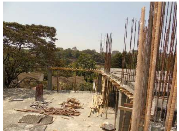
View of ground floor.
