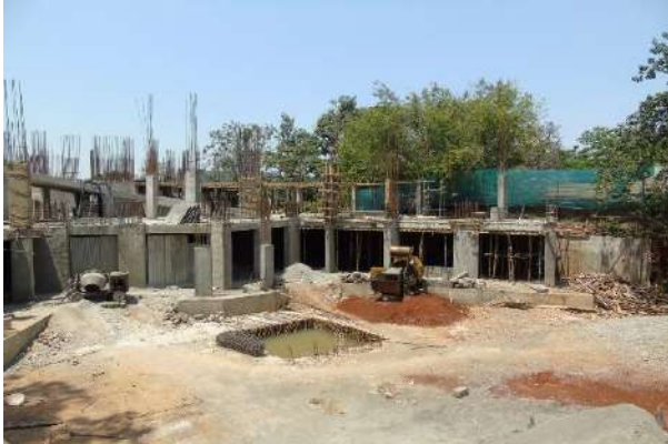
Structural elevation work on ground floor underway.
