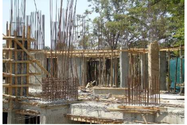
Concreting work on beam and column underway
