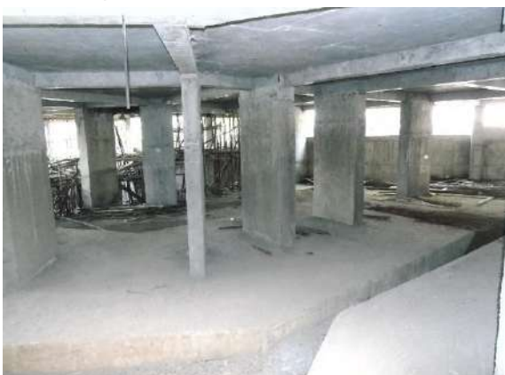
View of basement.
