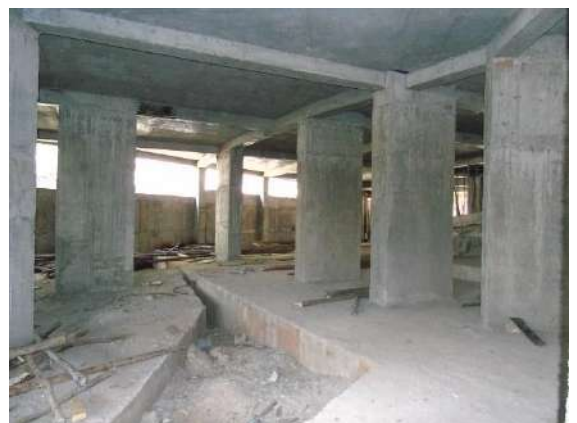
View of basement.
