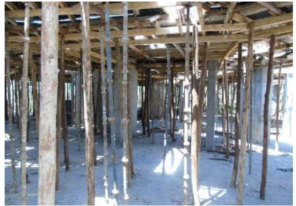
Structural elevation work for ground floor underway.
